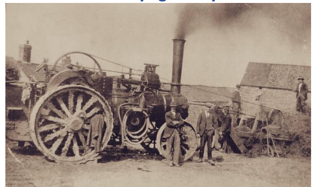
A steam engine at work at Tong's farm, Wrawby, hulling red clover. The Chaff Cutter is a Fletcher from Newport Iron Works Winterton .
